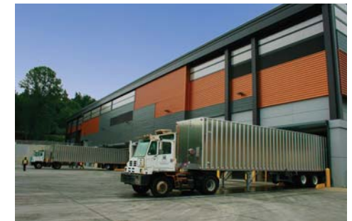
Work to replace the Factoria Transfer Station in Bellevue began in 2014 and is expected to be fully completed in late 2017.
